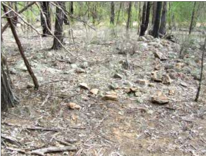
The south-west corner of a former large dwelling, now a pile of rubble flanked by former pathways.
